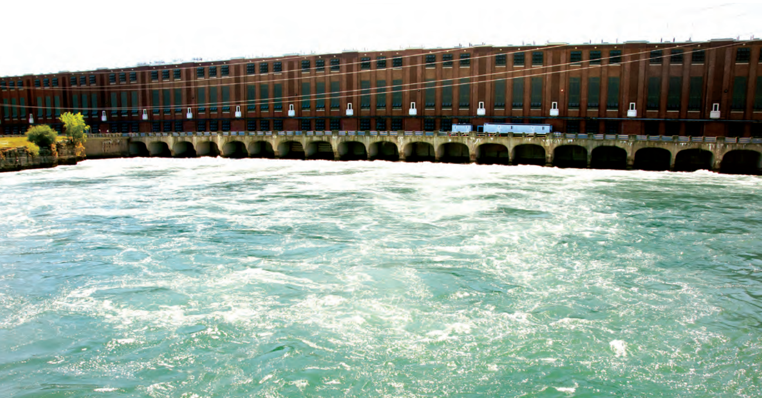
Progesys project: Beauharnois Hydroelectric Dam, Beauharnois, Québec, Canada
