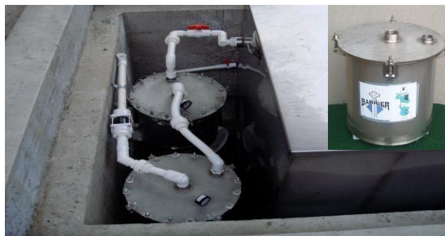
Polishing Filters for Removal of Heavy Metals and Oils. The Marine Guard P3 was a finalist for the 2008 VIATeC Award for Environmental Excellence.
