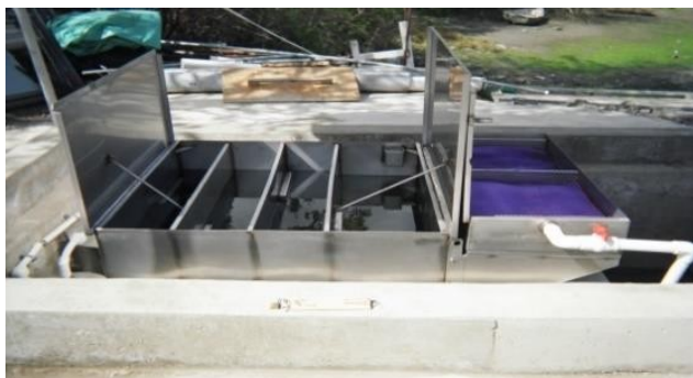
“OIL WATER SEPARATOR” Pre-Filter and Four Compartment Oil-Water Separator.
