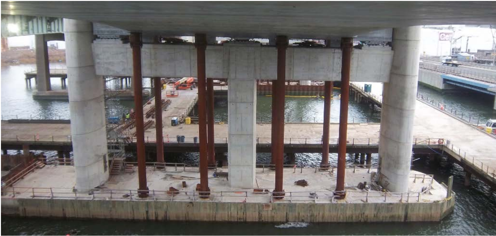
Temporary Structural Supports for Pearl Harbor Memorial Bridge in New Haven, Connecticut
