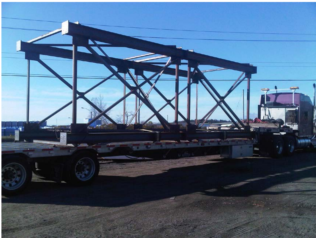
TEMPORARY BRIDGE SUPPOR TRUSSES
