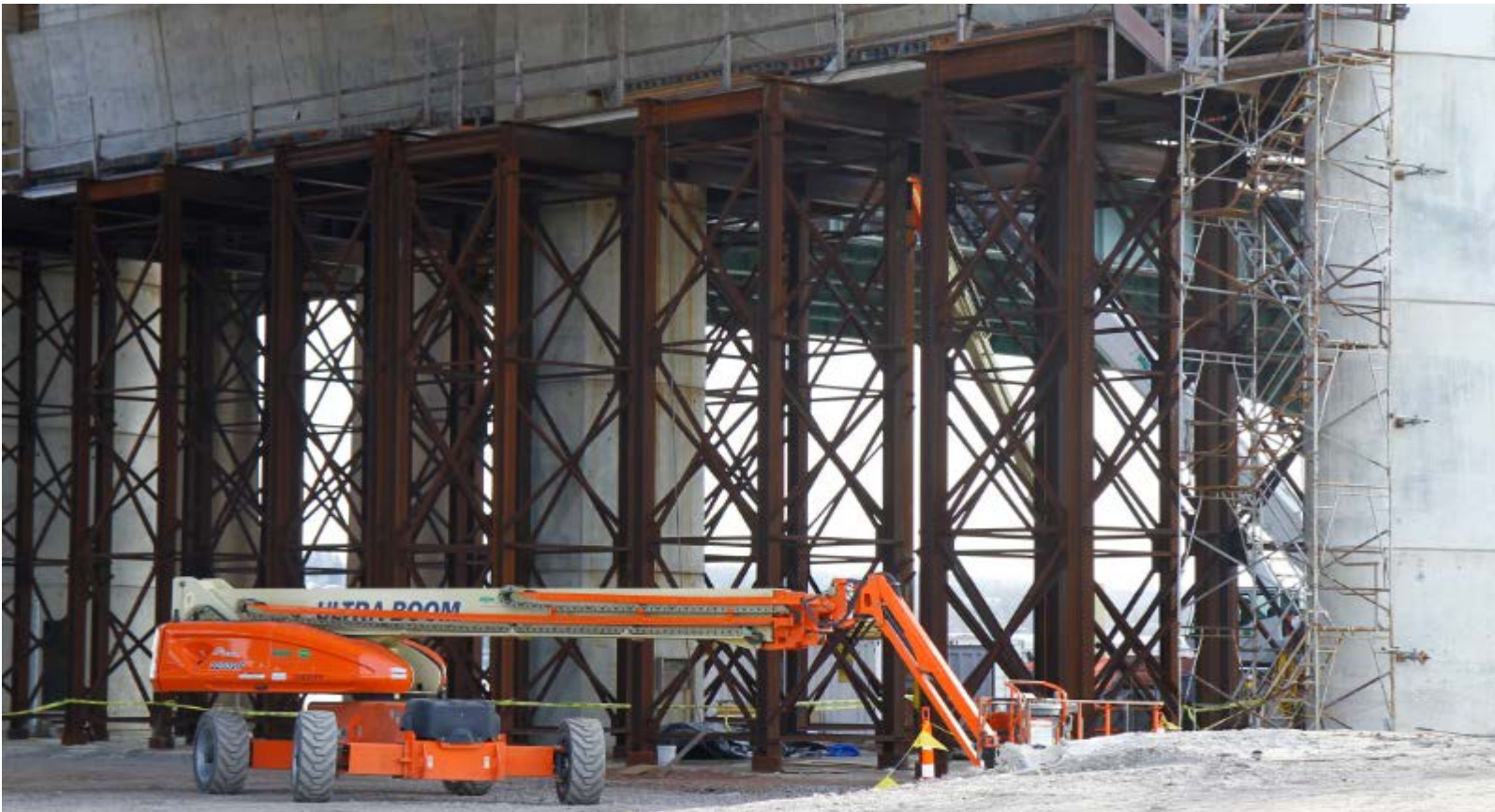
Temporary Structural Supports for Pearl Harbor Memorial Bridge in New Haven, Connecticut
