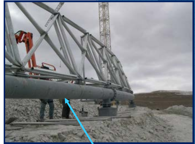
Perimeter Steel Tension Ring
