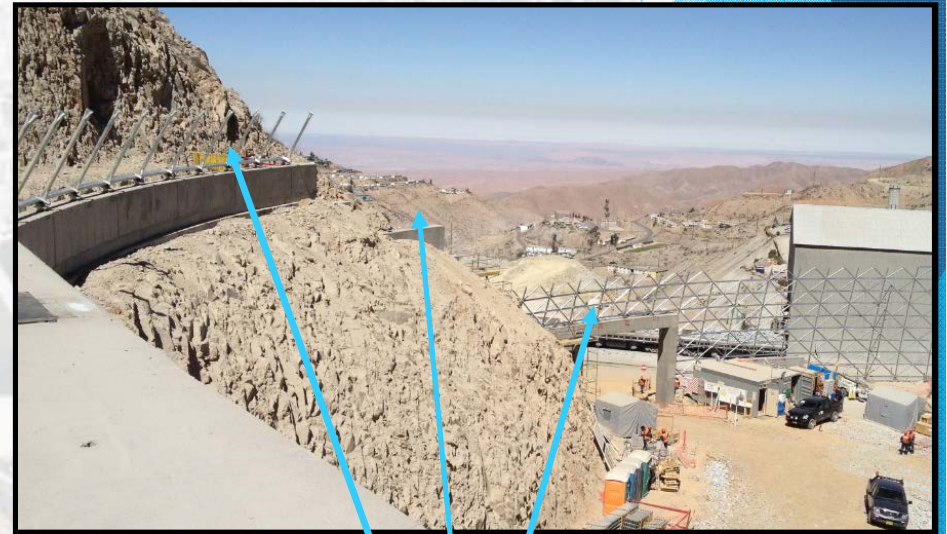
Dome Supports Ring 1 to 11 Concrete Foundation Wall
