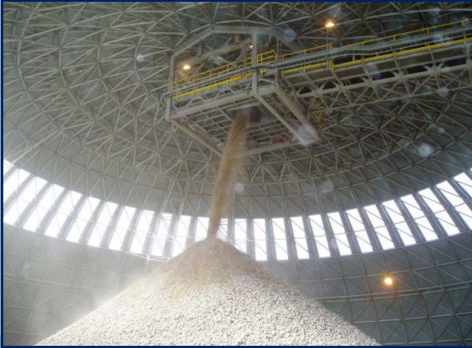
Veladero mine Argentina 55m diameter Dome supporting conveyor gallery Barrick Gold
