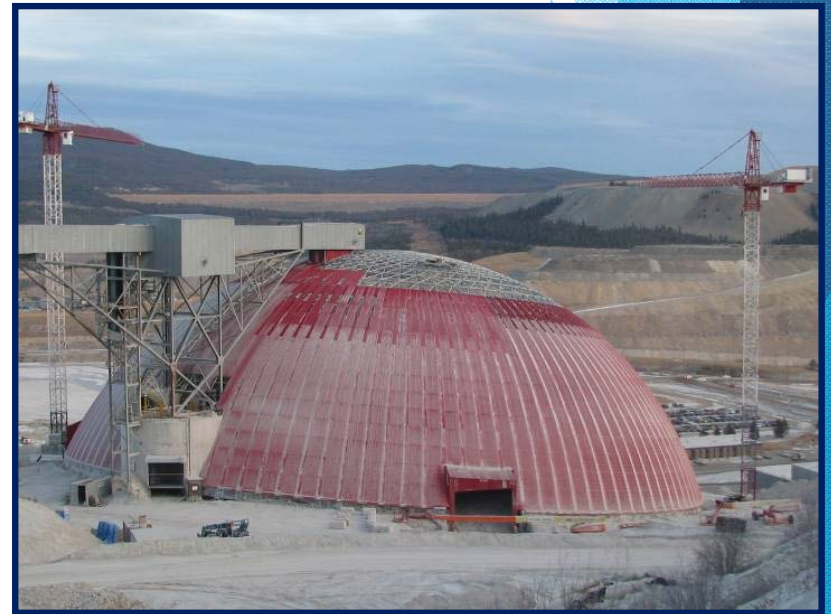
Perimeter Steel Tension Ring
