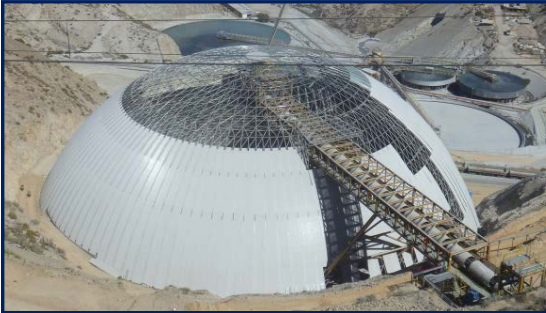
Toquepala Mine 115m Diameter Side loaded Dome
