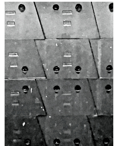
Taperline - Diagonal Liner Layout
