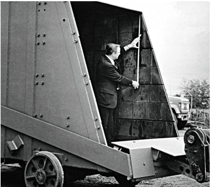
Don Wilding (original inventor) in a Domite Lined Blast Furnace Skip, material handled Coke & Iron Ore. Photo 1970
