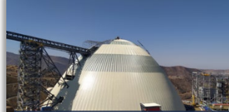
Quellaveco Mine, Anglo American D = 124m, Moquegua, Peru
