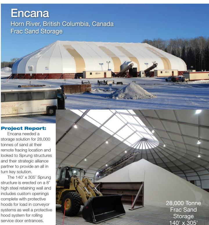
Sprung's exclusive radius end design provides an ideal configuration for sand storage which is much more space efficient.
