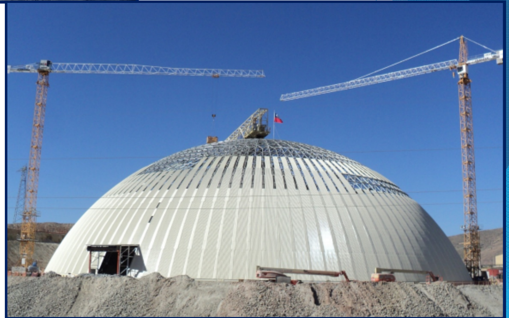
Andacollo Mine 98m Diameter Top loaded Dome
