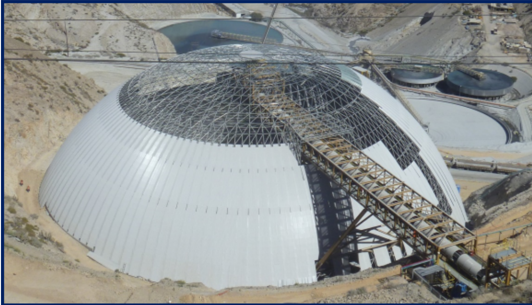
Toquepala Mine 115m Diameter Side loaded Dome
