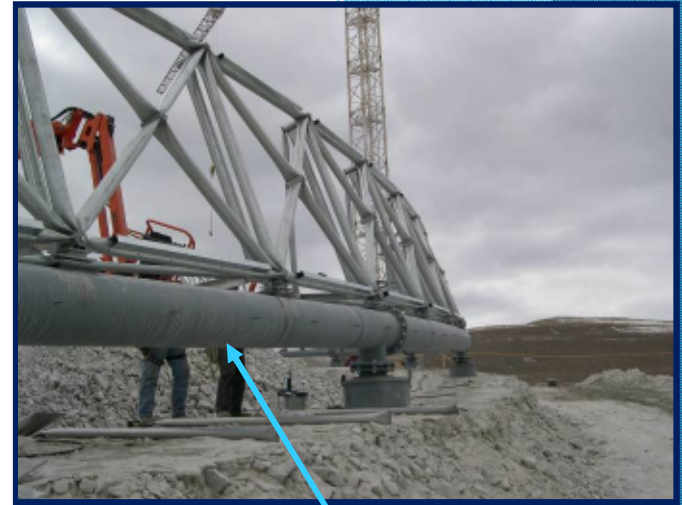
Perimeter Steel Tension Ring
