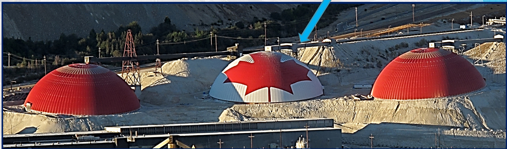
Highland Valley Copper mine B.C. 3 Domes 105 m diameter (top loaded) (One of the biggest Canadian Flag)
