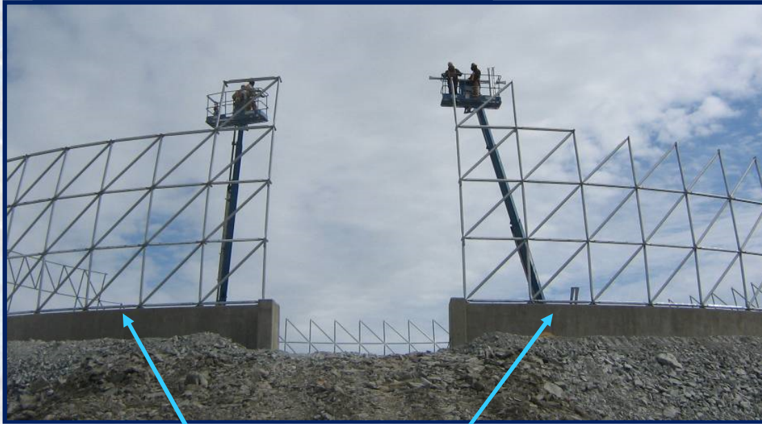
All Dome Supported at Ring # 1 Concrete Foundation Wall
